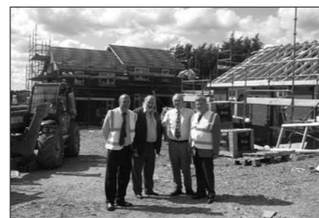
Board Members and Staff Inspect Kinallen Phase II
